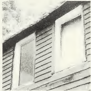
Window trim removed
